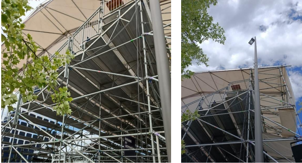
Figures 6 & 7 - Views of the grandstands and LED lights.
