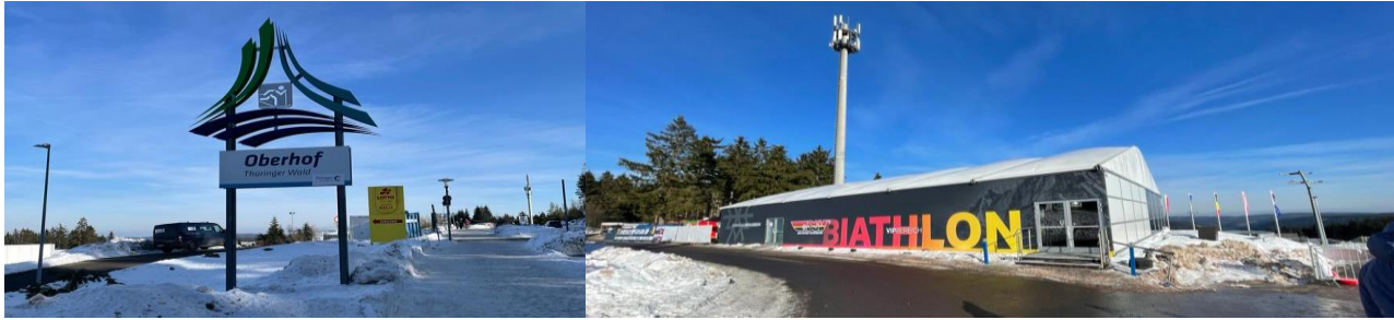
Figure 132- The entrance to the LOTTO Thüringen ARENA and the pavilion dedicated to the German Ski Federation
