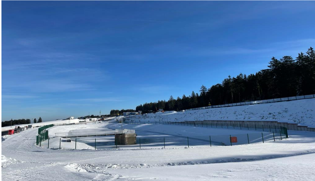
Figure 48 - (Rainwater) collection pond for artificial snow production
